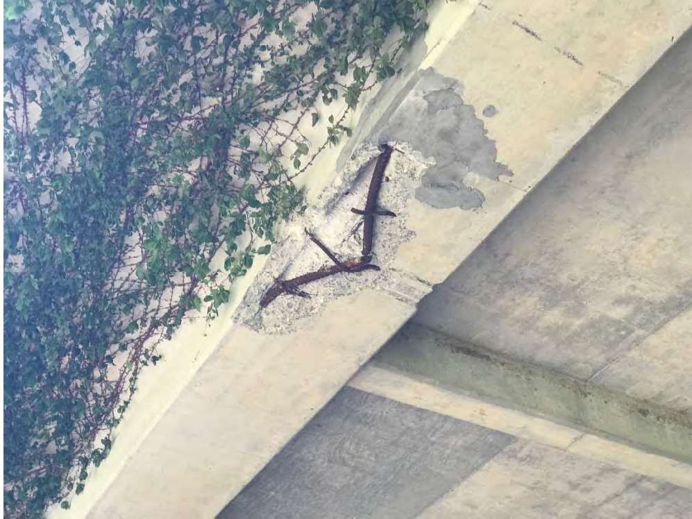
Closeup of damage under bridge
